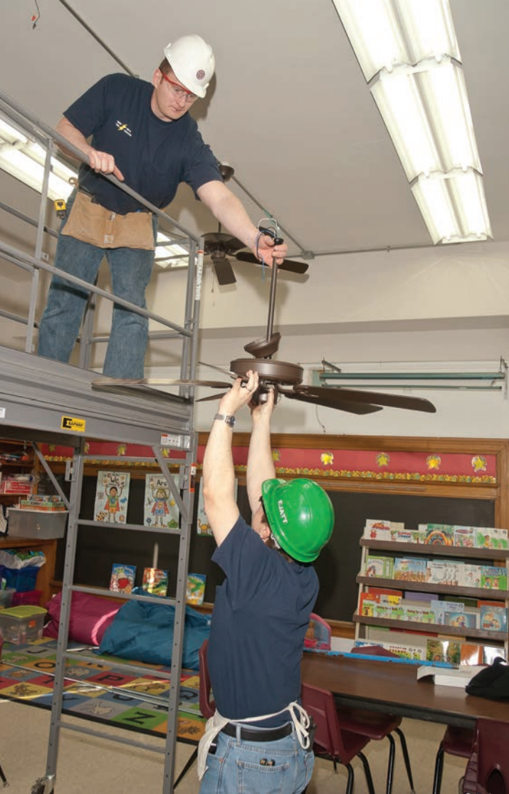
CLOCKWISE FROM TOP LEFT: CHRIS RAWSON AND MARK BERCHMAN OF IBEW LOCAL 134 INSTALL A CEILING FAN IN A CLASSROOM.
